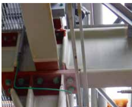
Intumescent fireproofing installed by certified applicators.
